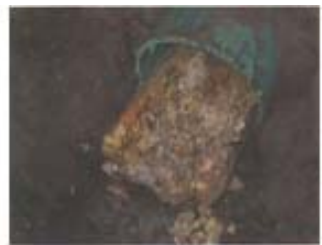
GREASE CLOGS REMOVED FROM RESIDENTIAL SEWER LINE
